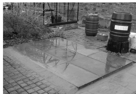
A 6x8 slab base: ideal for a 5x6 greenhouse. Remember that your greenhouse is a few inches bigger than the nominal size.
